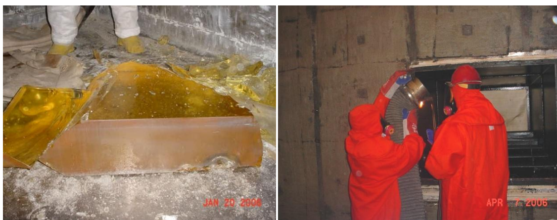
Figures 9 and 10. Removal of hot cell window glass and frame
