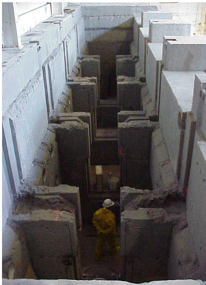
Figure 13. Decontaminated hot cells, with roof and intercell doors removed
