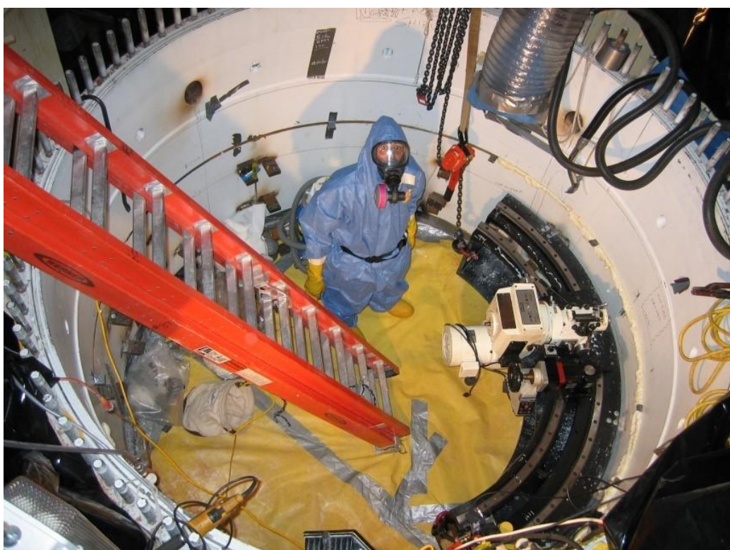
Figure 6. Segmenting the vessel with a milling machine
