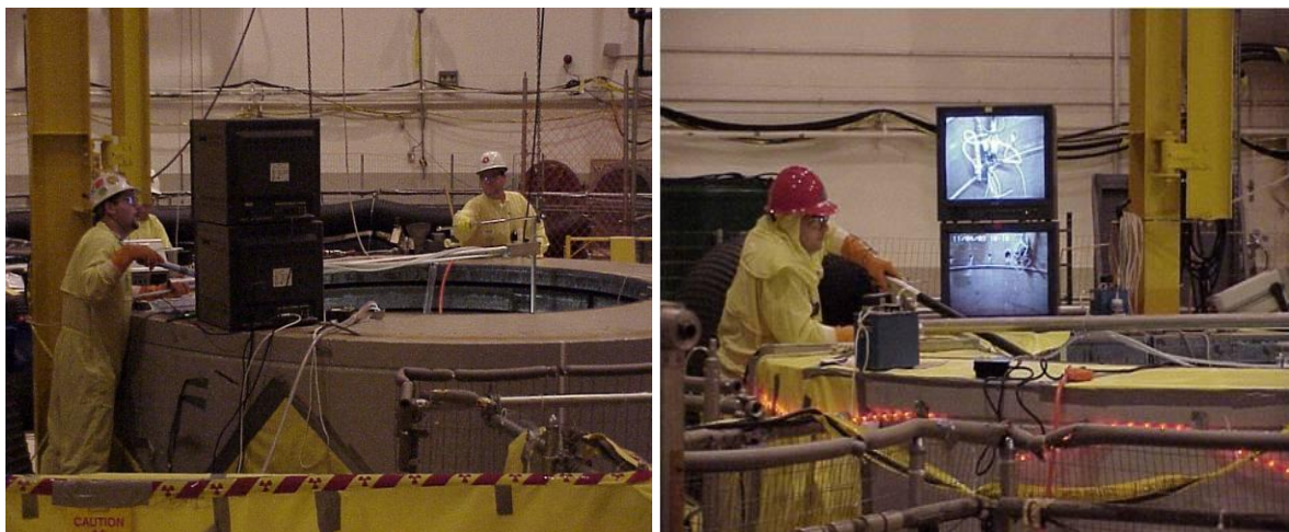
Figures 3 and 4. Workers using remote viewing and long reach tools
