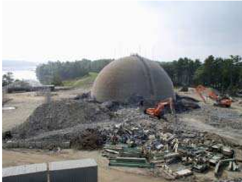
Figure 1. Demolition of Maine Yankee's Containment: Decommissioning is not Over Yet!!!
