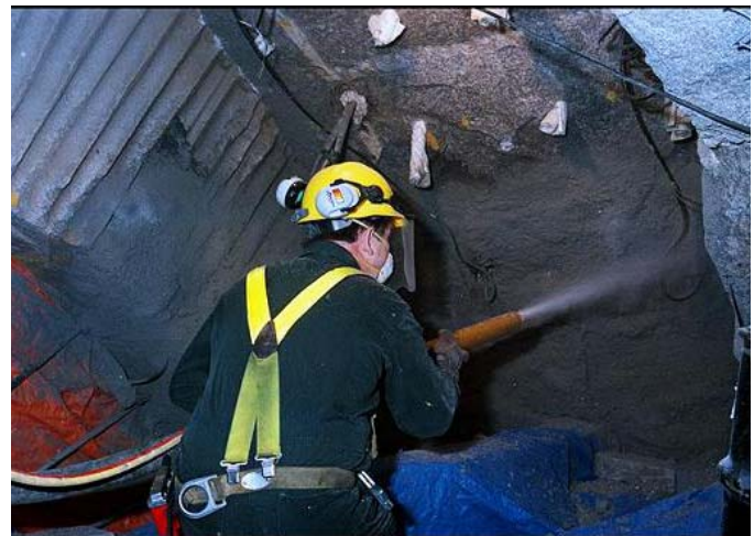
(b) Shotclay Application To Surface of Key
