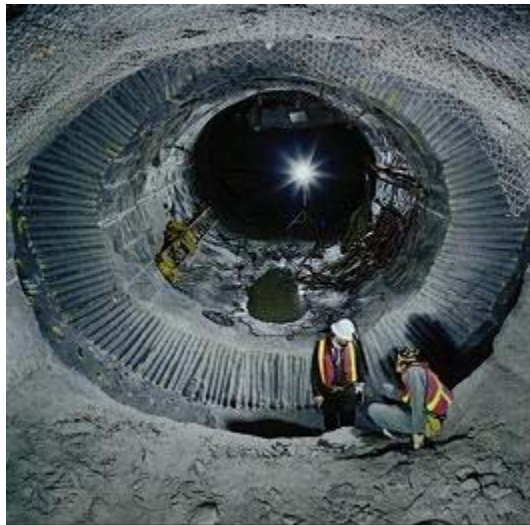
(a) Excavated Key for Clay Bulkhead
