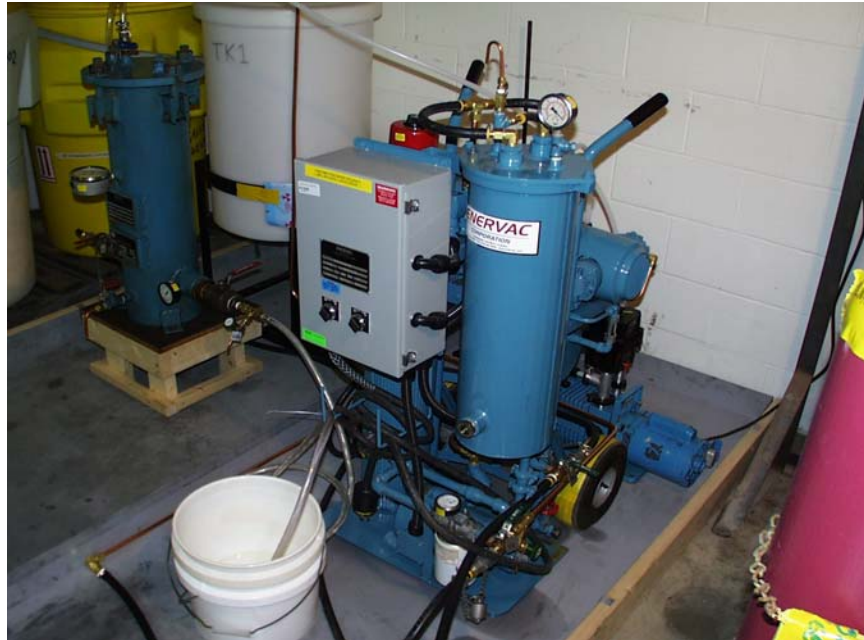
Figure 1 Oil Degassing Unit and Activated Alumina Cartridge
