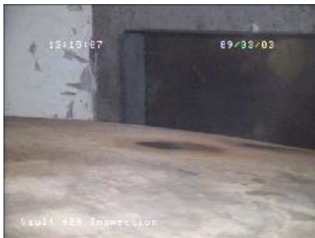
Figure 14: Rust Spots on the Outside of a Tank
