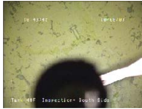
Figure 5: Debris Discovered in the Tanks
