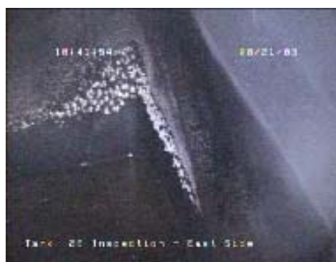
Figure 8: Sludge and Salt Build-up on Internal Tank Walls
