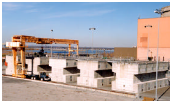
Figure III-1 Typical MACSTOR Dry Storage Module Site – Gentilly 2
