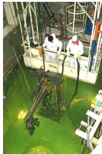
Pictures 1 and 2: The two main mechanical cutting techniques used for the dismantling of the reactor internals and the reactor pressure vessel
