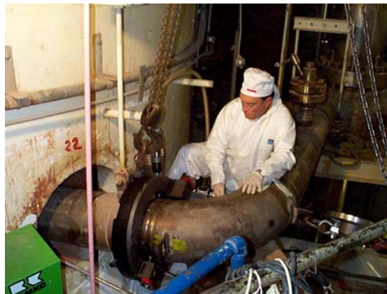
Photo 3: The cutting of the primary loop (cold leg) with a commercial pipe cutter
