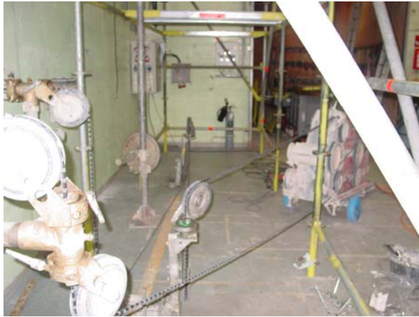
Photo 4: This is a view on the diamond cable cutting system used for the making of the opening in the spent fuel pool (the main dust collection system is situated on the other side of the wall and is not visible on the photo).
