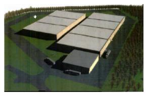
The Shielded Modular Above Ground Storage (SMAGS) structures are based on the same principle as the MAGS, with the metal wall replaced by a 10-inch concrete wall. The SMAGS structures will house the MAGS type waste and some higher activity wastes from the bunkers. The SMAGS provides better use of available land. A project is currently underway to begin construction the first on these structures in 2006.
