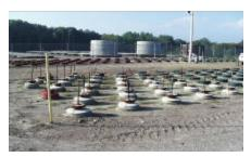
Tile holes are concrete, steel-lined containers intended for high-level waste. Tile holes are 3.6 to 4.9 m deep and from 15 cm to 90 cm wide. The excavated tile hole construction area is backfilled with sand.
