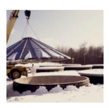
While in use, the bunkers are covered with a metal weather shield. On closure, the bunker is covered with a flat 6 inch reinforced concrete roof.
