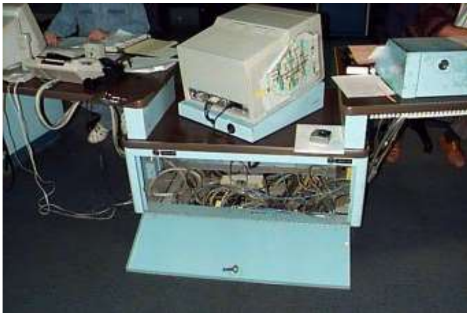
Figure 5 : Central Console Termination Rack Pre Change-out.
